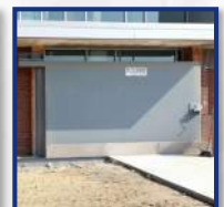
Sliding Flood Barrier
