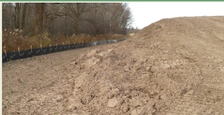
Silt fence around a soil stockpile.
